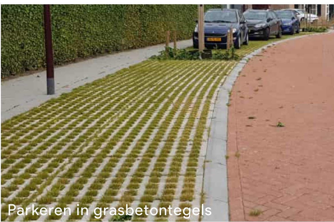
Parkeren in grasbetontegels
